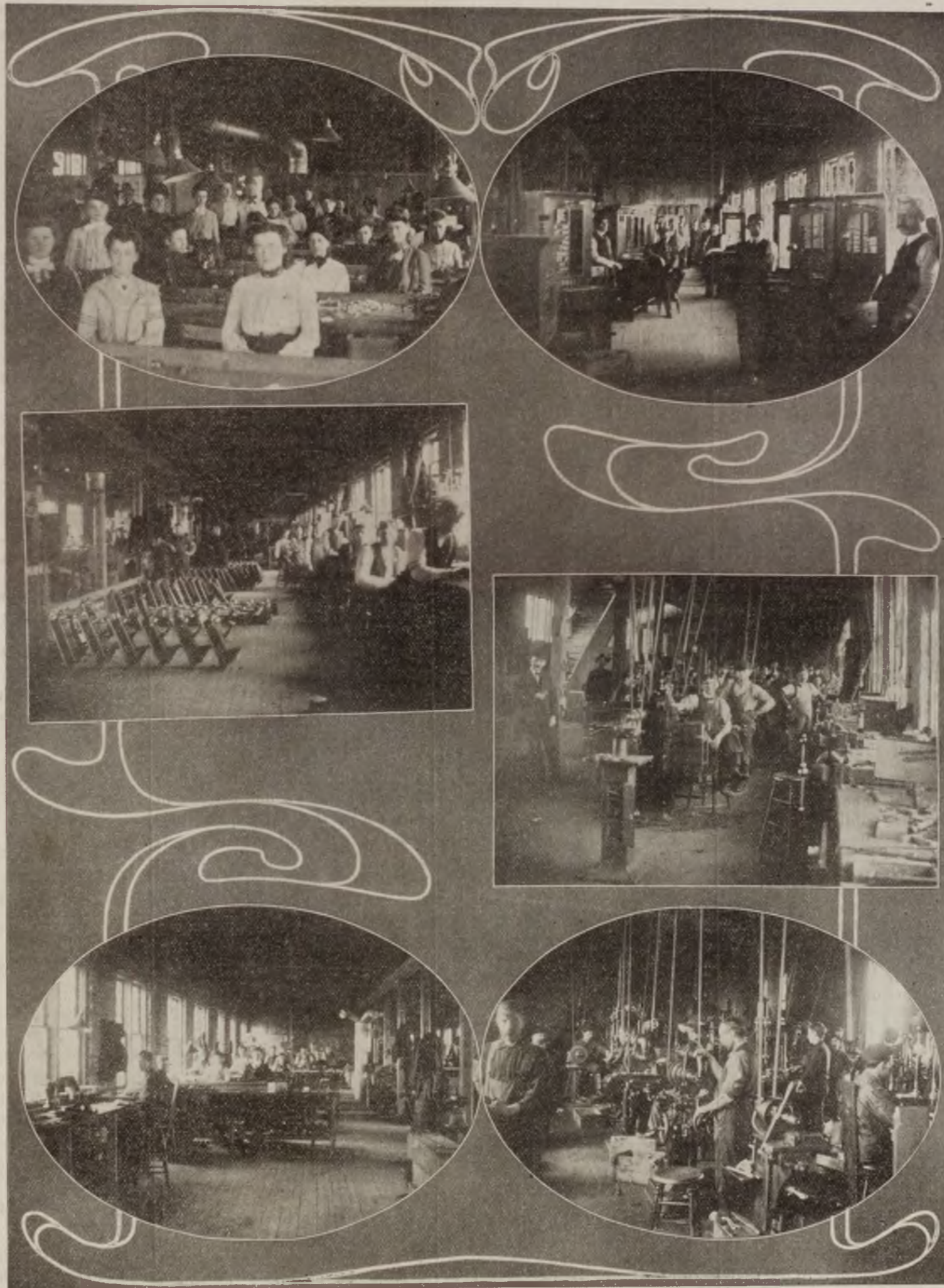
Views in the Eureka Electric Company's Factory, Genoa, Illinois
