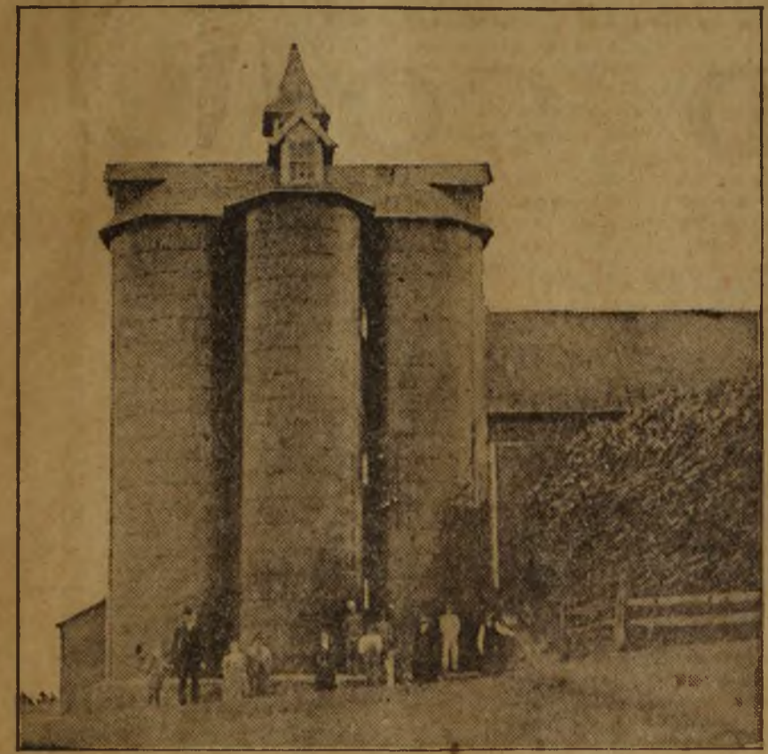
Modern Cement Silo on Fernwood Dairy Farm, Royersford, Pa.
