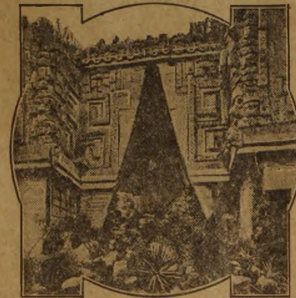
WEST FACADE OF GOVERNOR'S PALACE
