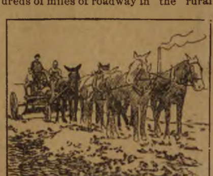
Slag Foundation and Broken stone Surface.
