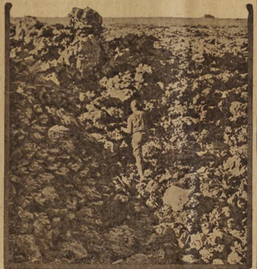
Ground Pulverized by Bursting of Big Shells.
