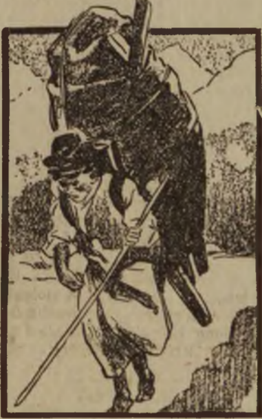
Material Carried Up.
