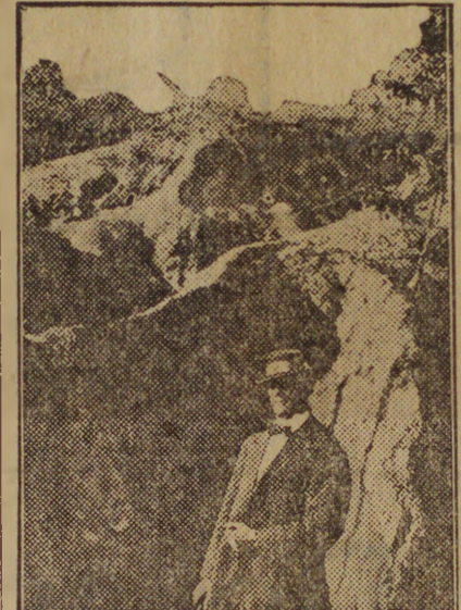
Bad Erosion Results From Clearing Land of Too Steep Slope.
