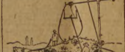
Derrick for Loading.
