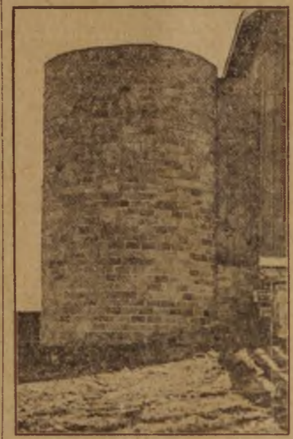
New Tile Silo at Iowa State College
