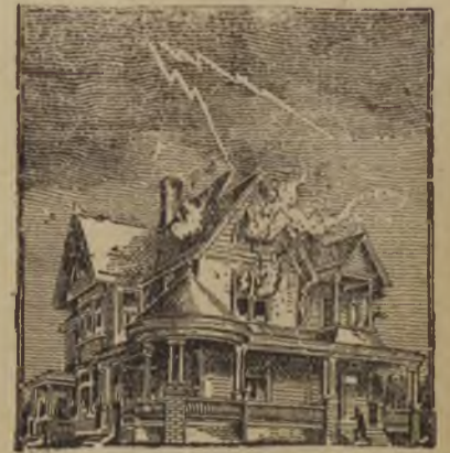
No protection here
