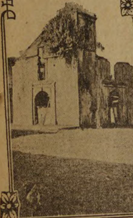
Remains of The Old Church at Porto Bello.
