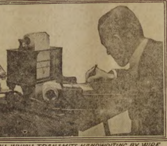
THE TEL-AUTOGRAPH WHICH TRANSMITS HANDWRITING BY WIRE
