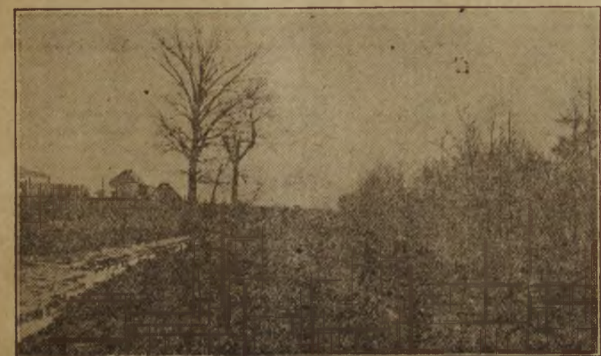
A road that is undrained, undragged, useless and uninviting. Query: Is it a highway or mireway? The march of progress over such roads will certainly be slow. Such roads mean isolation, drudgery, poor schools, poverty and wretchedness. The building of good roads will practically double the value of such farm lands and the State and Federal Government ought to help build the roads. A good road ought to change the name of such a locality from Mud Flats to Pleasant Plains.
