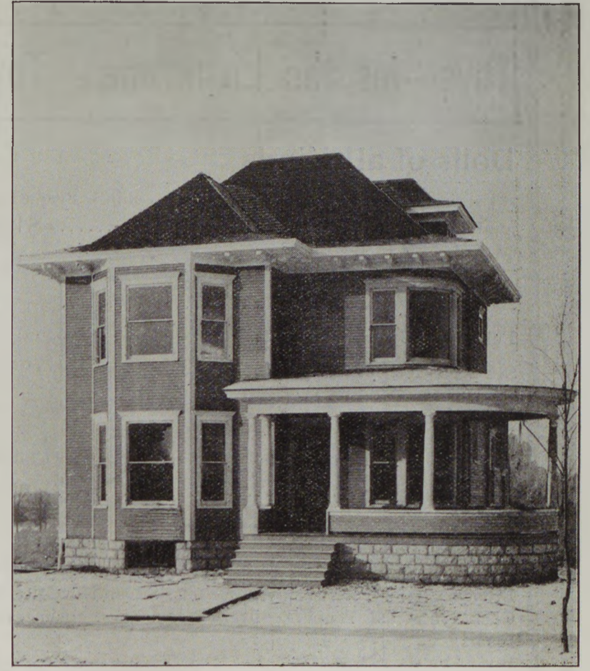
Residence of H. A. Kellogg In the Moan addition. Built by Jas. J. Hammond.
