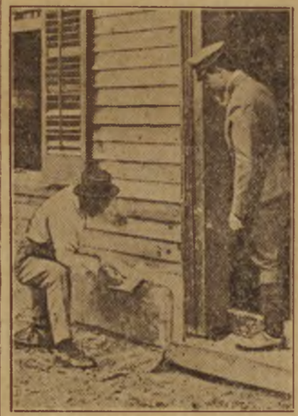
Putting in Cement Foundation.
