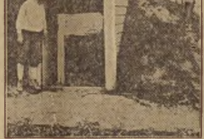
An Outdoor Storage Cellar, Built Partly Underground, for Storing Garden Vegetables. It Is Built of Concrete Except the Entrance, Which Is Frame, and Is Frost Proof. Where the Cold Is Not Severe Less Protection Than Is Shown Here Is Needed.
