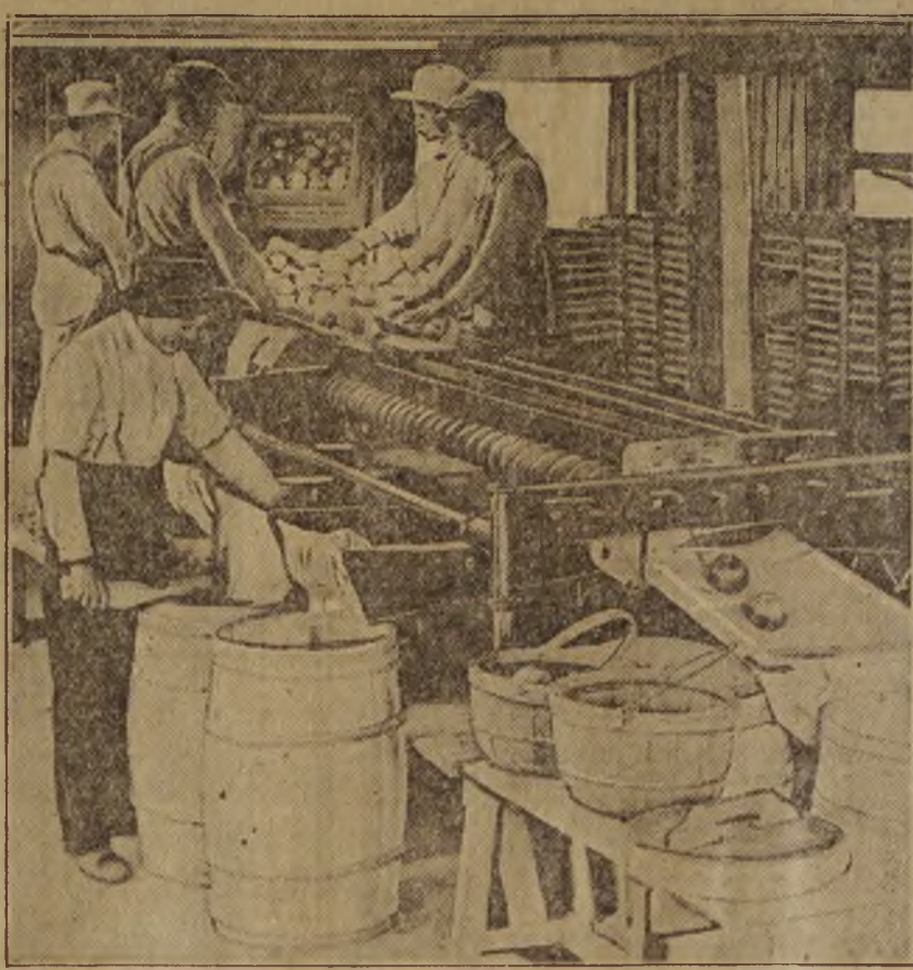
An Apple Sizer and Grader in Operation.
