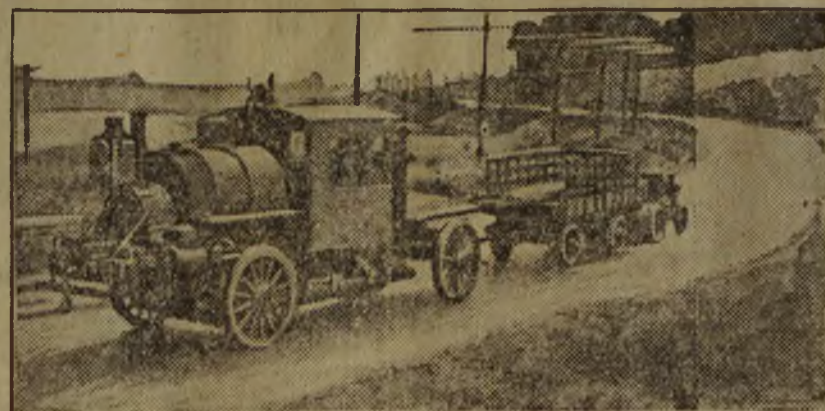
Motor Truck Pulling an 18-Ton Engine Between Los Angeles and San Pedro, Cal.
