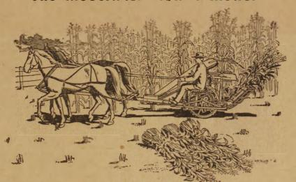
Is the only mower that gets all the grass. It is a very easy matter for a poorly constructed machine to run over a dollar's worth of grass on an acre, leaving it in stubble where it is lost. It is the only mower with a draft rod extending from the inner shoe to the shifting doubletrees.
