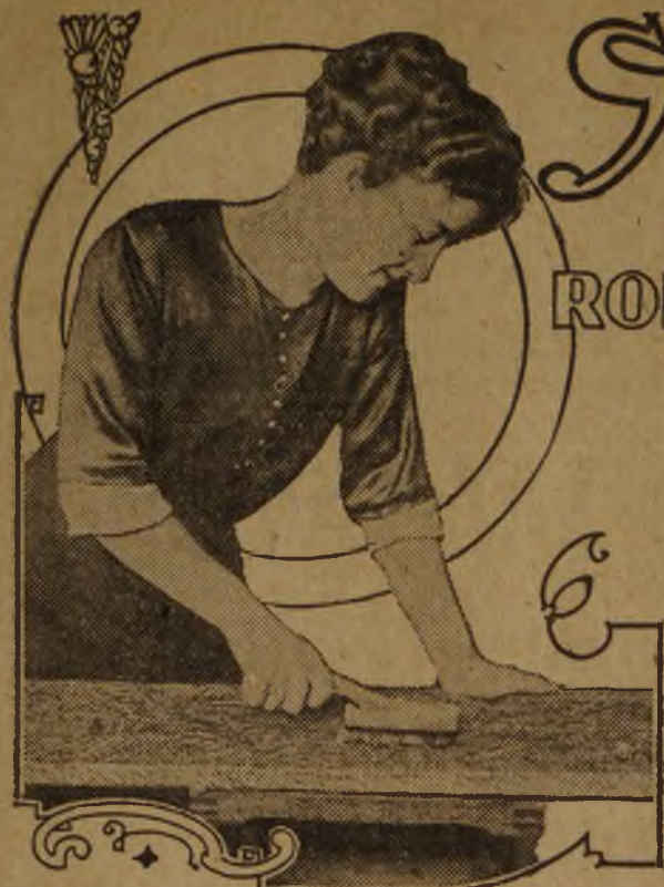
AFTER THE CYPRESS IS BURNED IT IS RUBBED WITH A STIFF BRUSH
