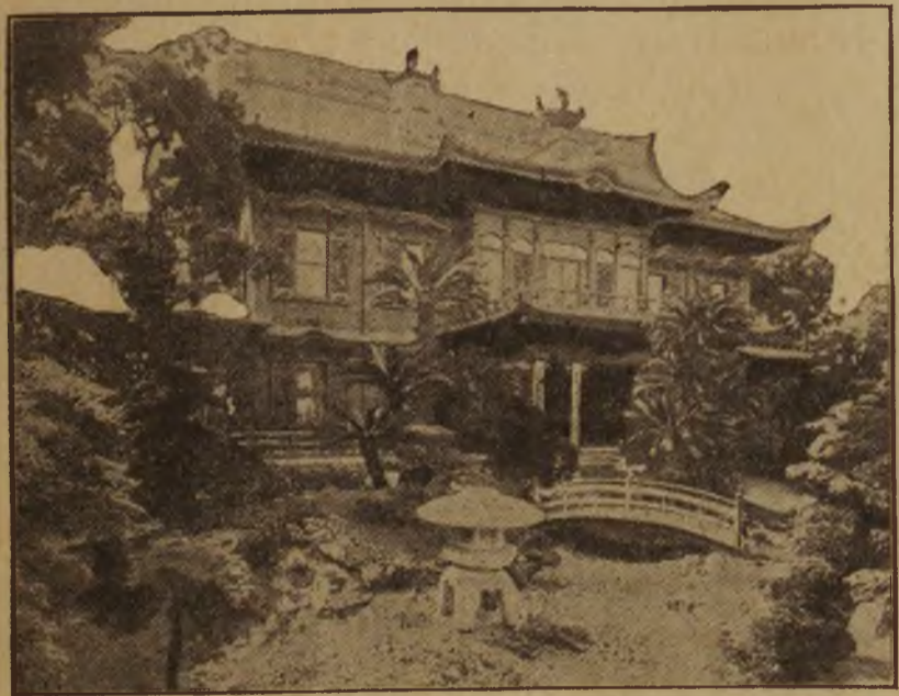
The Roof With the Devil in It. (The Devil Around Corner to the Left Cannot Be Seen.)
