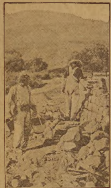
Construction of Cobblestone Masonry Wall.
