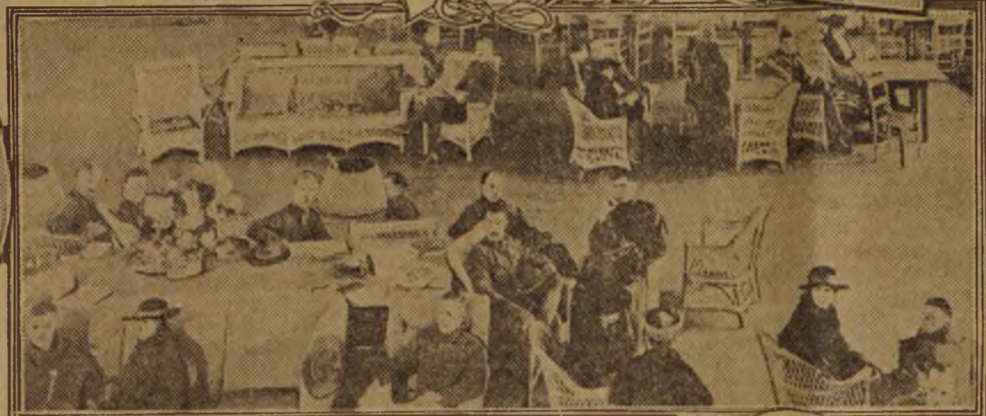
INTERIOR OF HOSTESS HOUSE, CAMP LEWIS, WASHINGTON
