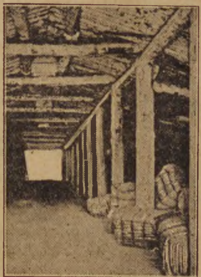
Interior of Satisfactory Potato Storage House With Earthen Side Walls.
