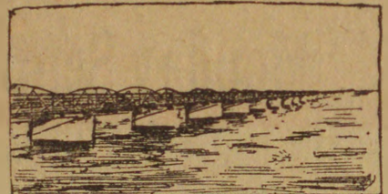
BRIDGE OVER GALVESTON BAY.
