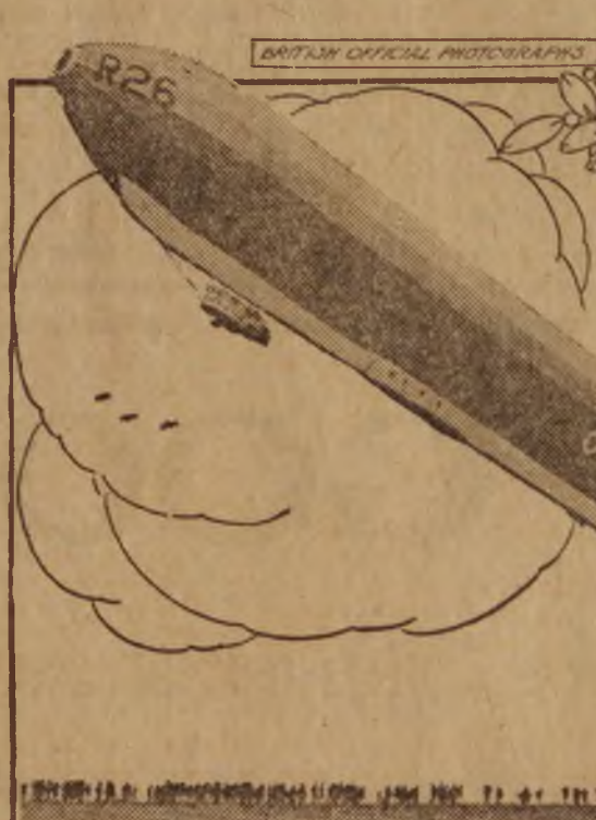
DIRIGIBLE NOW BUILDING TO HAVE TEN TIMES GAS CAPACITY OF THIS BIG AIRSHIP
