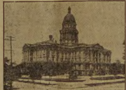
Colorado State Capitol Building, Denver.
