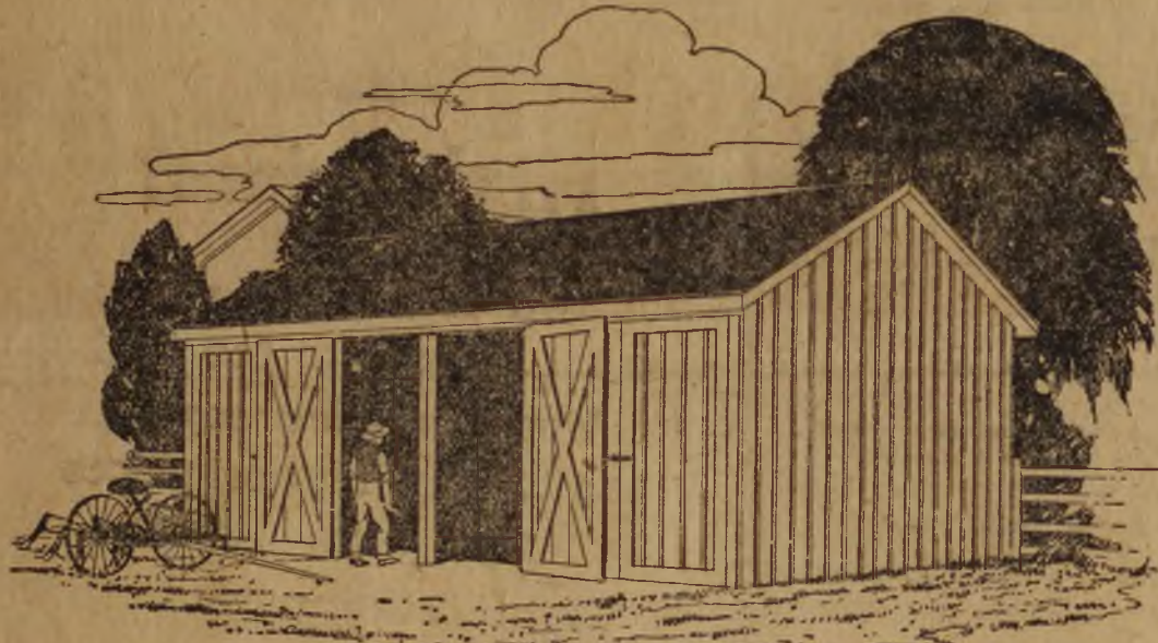
The FOUR-WALLED RECTANGULAR IMPLEMENT SHED Finished with White Pine Barn Boards and Battens
